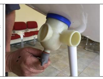
Assemble the new hose and manifolds to be placed on the cone. Ensure all clamps are done up tight.
